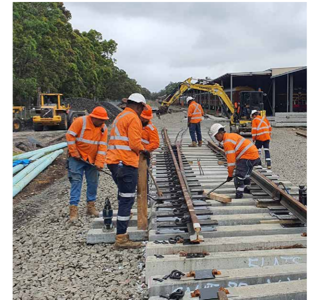
▼ Construction underway at Thirlmere B Frame.
