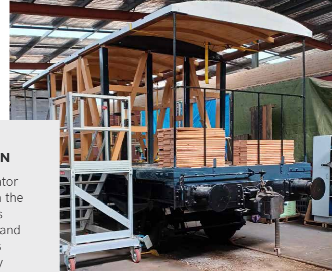
◀ Guard's Van CHG 16995 under restoration.
