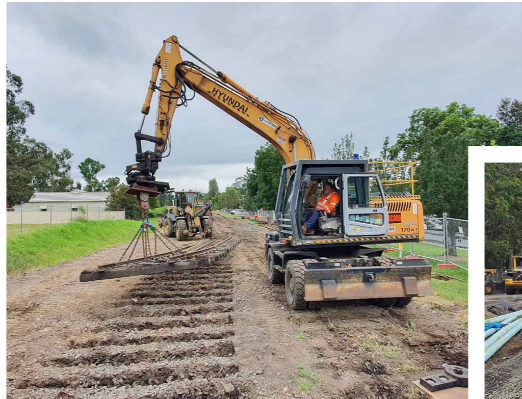
▼ The old Thirlmere A Frame is removed.
